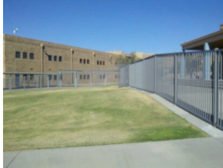
Installed fence panels at east side of La Cima campus
