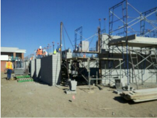
Exterior CMU wall installation MPR demo and new kitchen / serving line work
