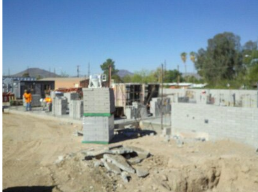
exterior block walls
