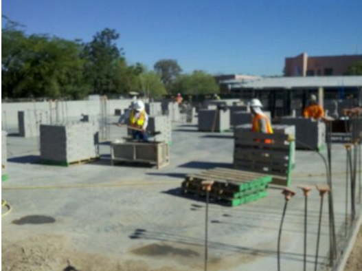
new building S.O.G.
