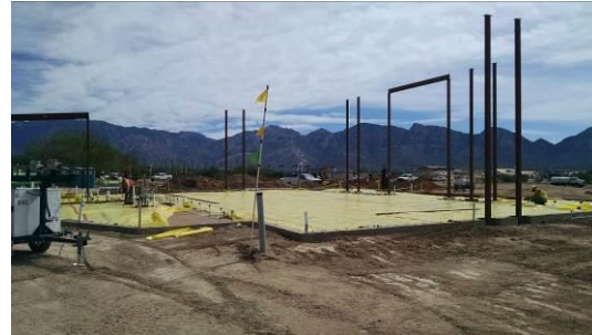
Vapor barrier at 100 building
