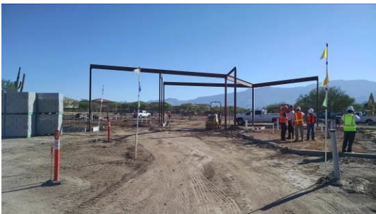
Steel erected between 100 & 200
