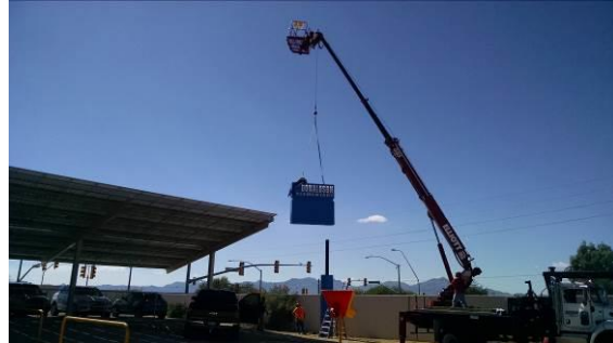
New Marquee Being Installed
