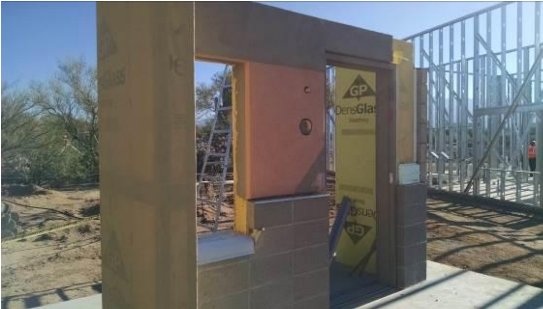
Mock-up of wall construction
