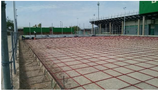
Tennis Court Post-tension Work
