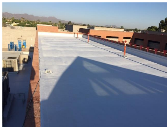
Keeling Administration Roof
