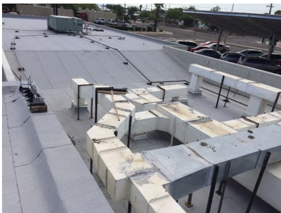
Roof at Keeling Annex
