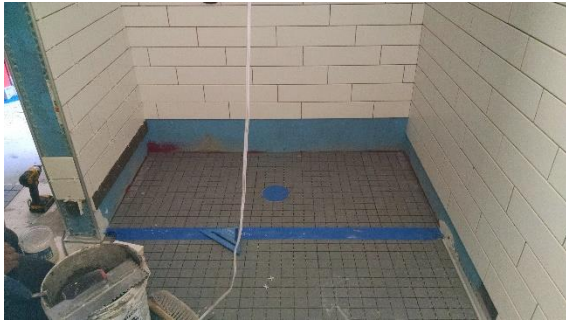
New Shower Area
