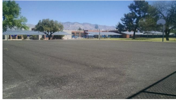
Ready for striping
