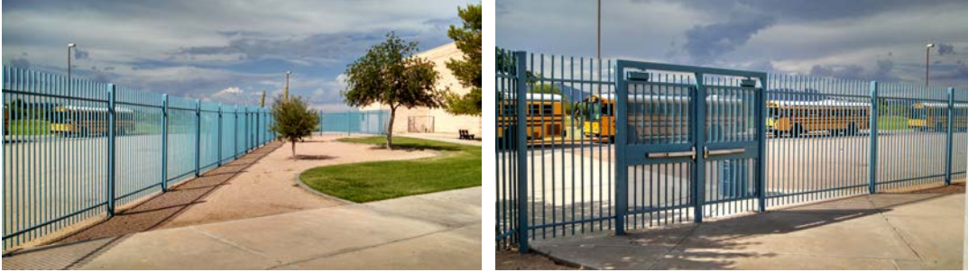
New Security Fence and Pedestrian Gates
