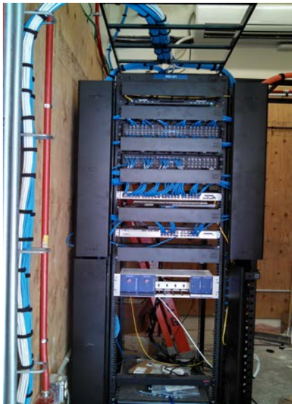
New IDF (intermediate distribution frame)
