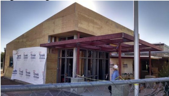
HR Dry-In and Interior MPE Rough-In
