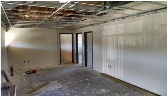
School Operations Offices – Painting, Ceiling Grid Installation, HVAC Above Ceiling Duct Installation, and Lighting Installation
