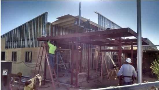
HR Framing and Structural Repairs
