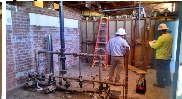
West Restroom Demolition East Restrooms Are Open (temporary doors and partitions)
