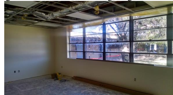
School Operations Offices – Painting, Ceiling Grid Installation, HVAC Above Ceiling Duct Installation, and Lighting Installation
