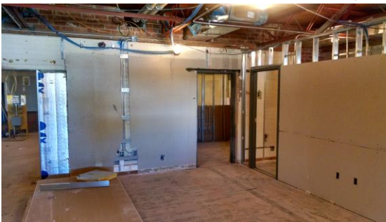
Technology Office – Drywall Installation, Insulating, and HVAC Rough-In
