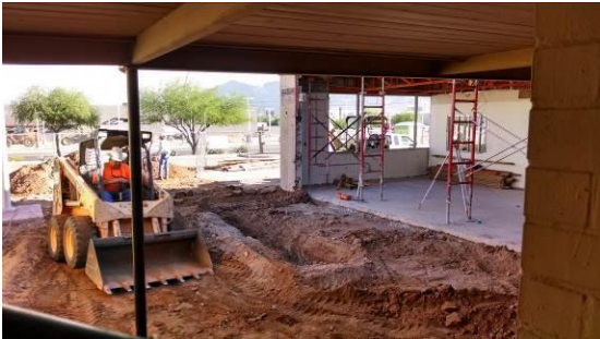
HR Office Addition Excavation
