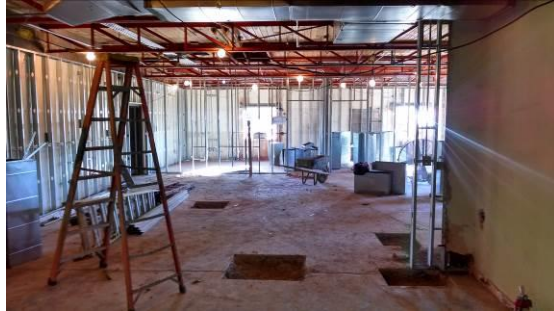
Federal Programs Framing and Electrical Rough-In
