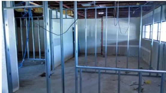
Technology Wing Framing, Electrical Rough-In and HVAC Modifications
