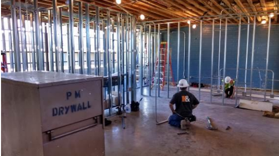
School Operations Offices Framing, Electrical Rough-In and HVAC Modifications
